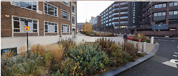
Figure 16.11 Grey to Green Phase 1 (Bridge Street): before and after (images from Google Streetview)
