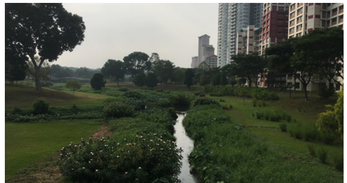
Figure 1.9 Sustainable drainage system, Bishan-Ang Mo Kio Park, Singapore
